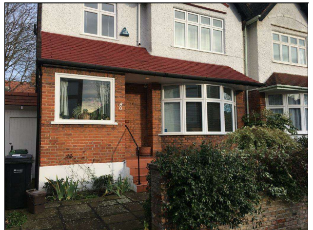
Front of property
