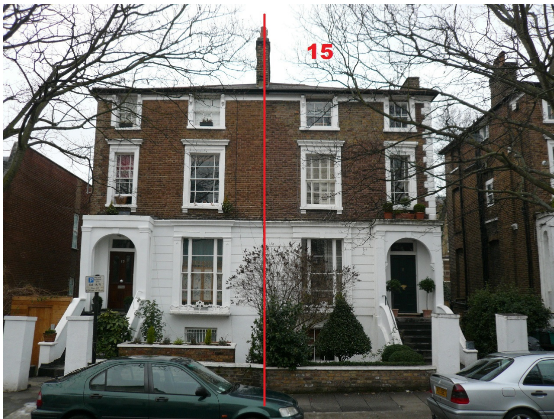
General view of the front elevation of number 15 Priory Terrace
