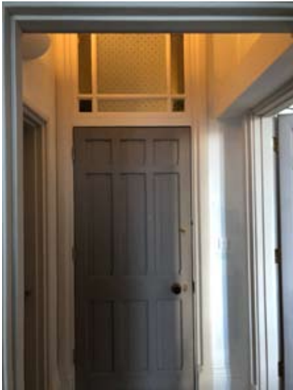
Entrance Hall - North elevation showing the main entrance door and surrounding framework.
