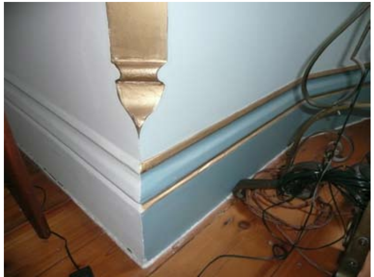
Room 3 - Plaster skirting detail .
