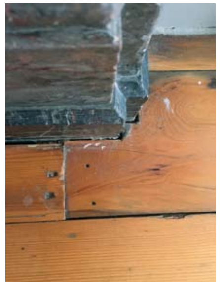
Detail of the flooring around the fireplace
