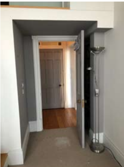
Room 1 - showing the doorway to the entrance hall with the threshold transition between the carpeted chipboard and the original softwood flooring.
