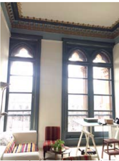
Room 1 - South elevation showing the original facade windows.
