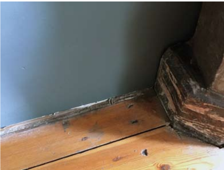
Detail showing the mastic used around the board covering the fireplace in Room 2
