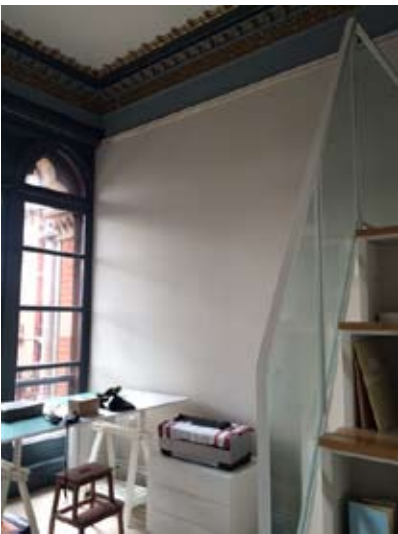
Room 1 - showing the west elevation.
