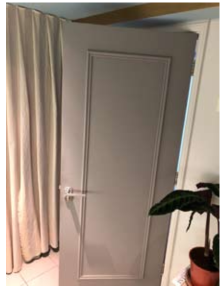
Bathroom - East elevation showing the door through to the entrance hall.
