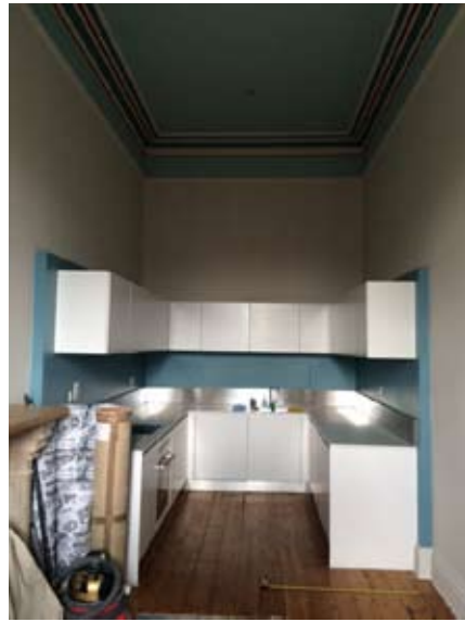
Room 3 - North elevation showing the side sub-walls to house the kitchen services
