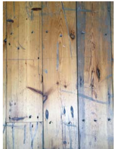
Detail showing the general marking and scuffing and nail holes
