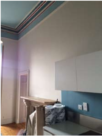
Room 3 - West elevation
