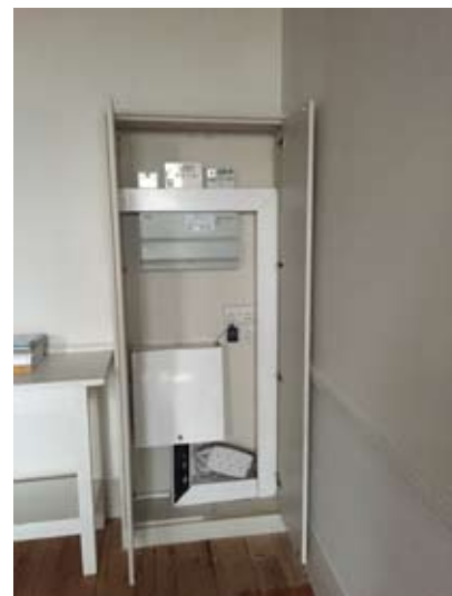
Room 2 - MDF cupboard currently installed to house the electrical provision for the apartment.
