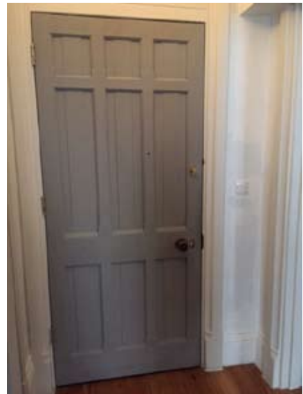
Entrance door - showing the door style of the existing original doors .
