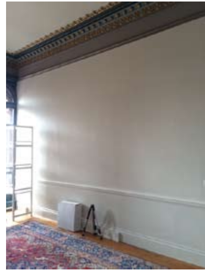
Room 2 - West elevation
