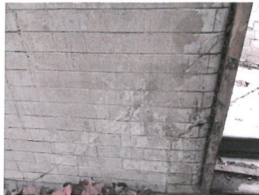
Severe cracking either side of entrance door, structural as well as cosmetic repairs required
