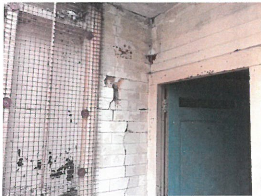
Severe cracking either side of entrance door, structural as well as cosmetic repairs required
