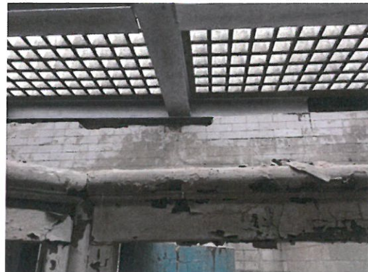
Missing and damaged tiles at high level following reinstatement of new roof light
