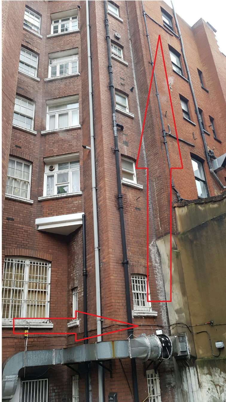
Extractor at Humaira Restaurant vented correctly above roof line, motor housing stood away from the building.
