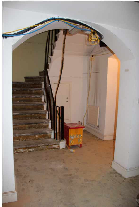
EXISTING CONDITION Structural opening
