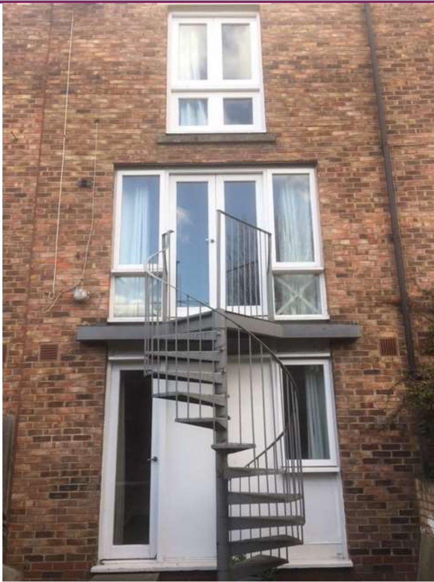
Figure 2 - Existing Rear Fenestration, 21 St Paul's Mews
