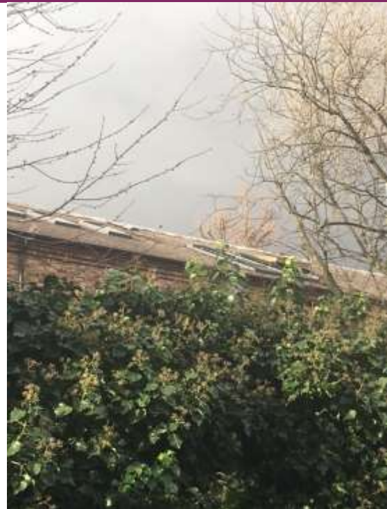
Roof Lights along St Paul's Mews
