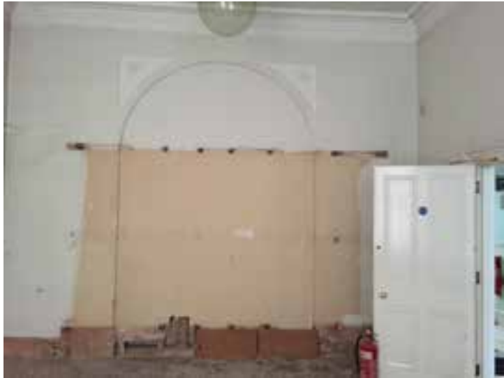
View of original opening to room G14 blocked in
