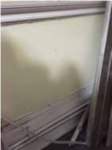
Detail of the moulded dado and skirting
