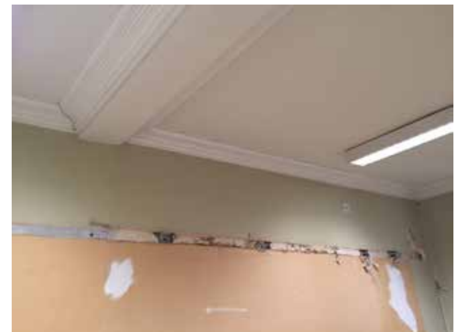
Views of ceiling showing down-stand beam which may be line of earlier wall
