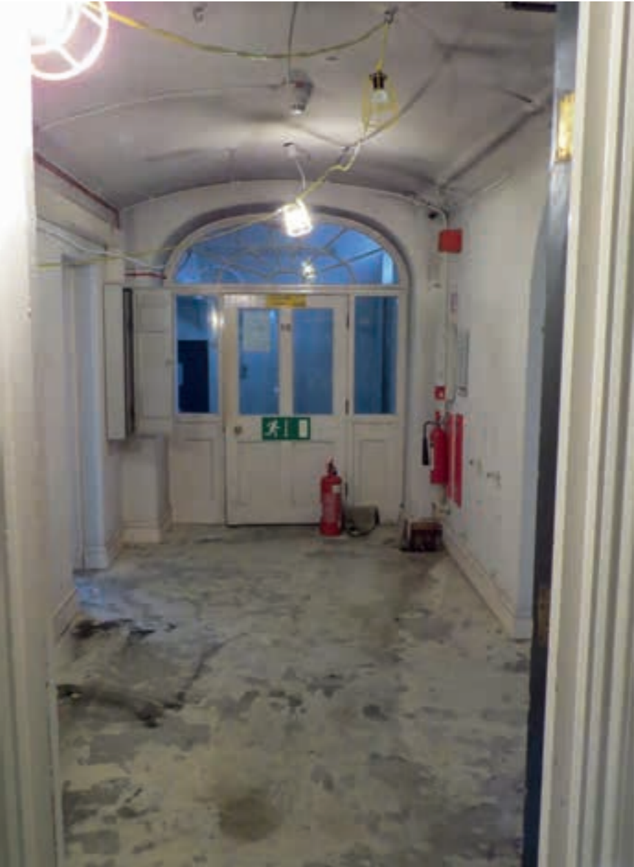
Figure 4.7 Fanlight at basement level
