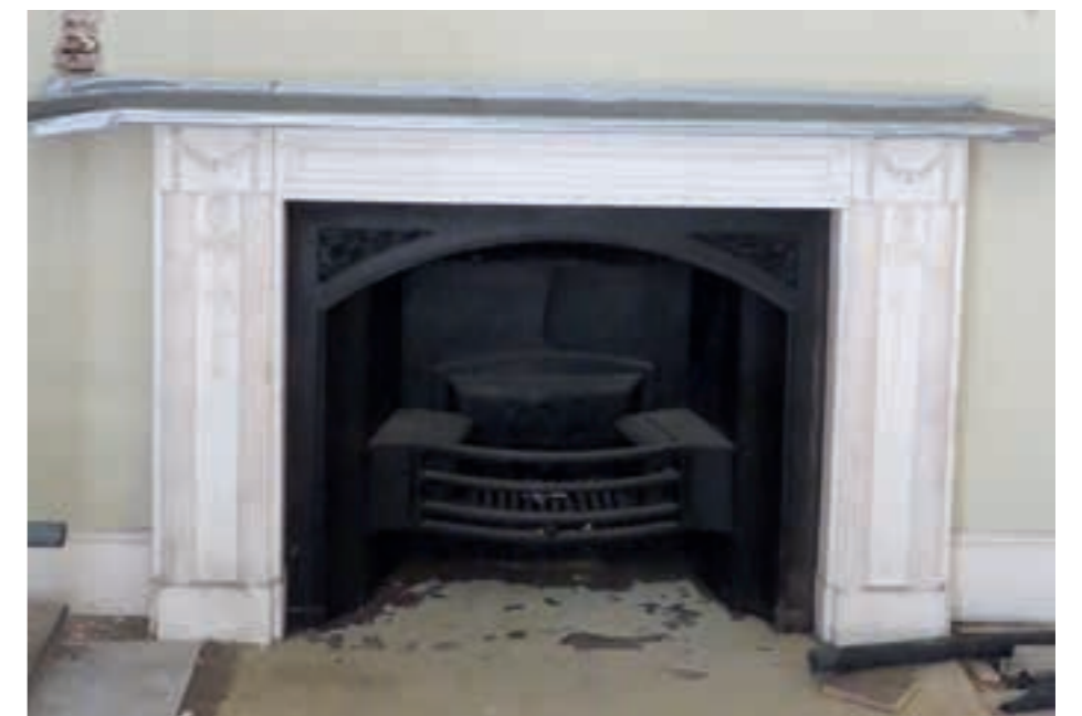
Figure 4.19 Marble fire surround with inset at first floor
