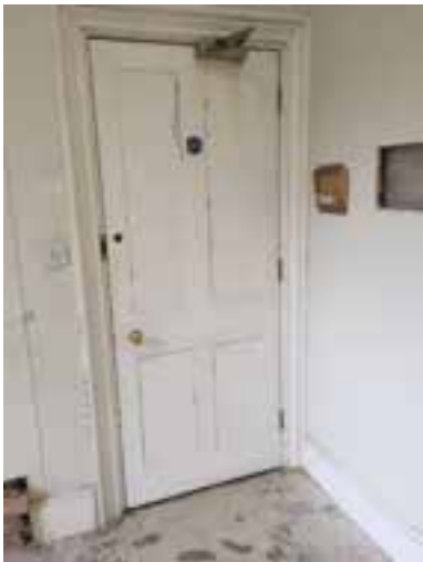
View of door to stairs with fire protection overboarding
