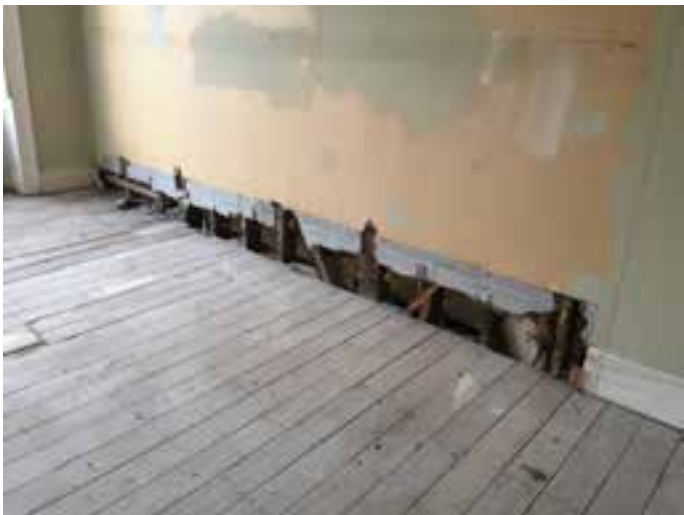
View of timber studs visible following removal of display cases
