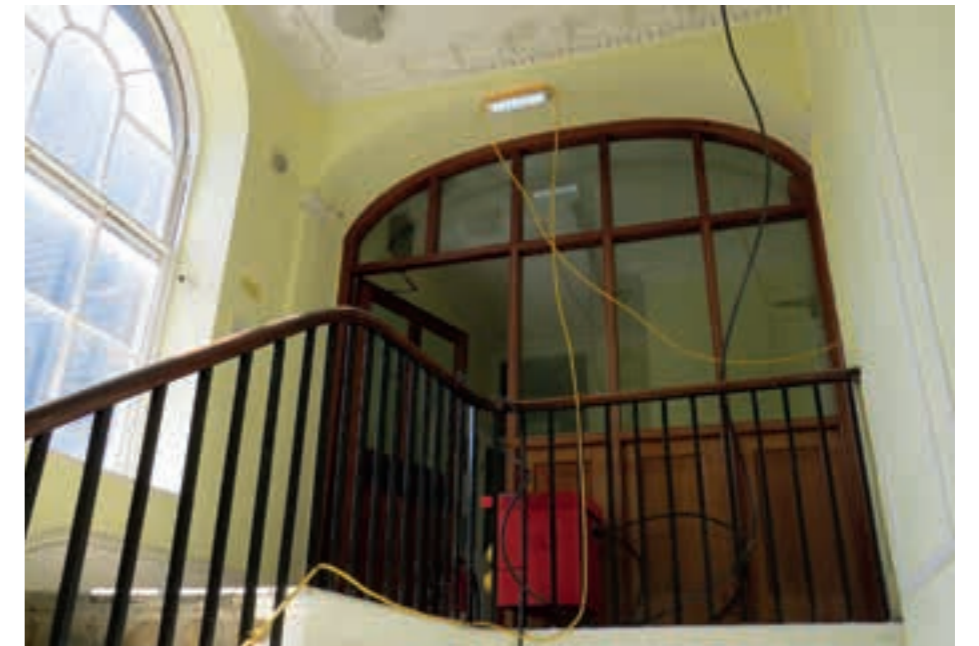
Figure 4.18 Staircase to no. 1, showing simpler balustrade and handrail
