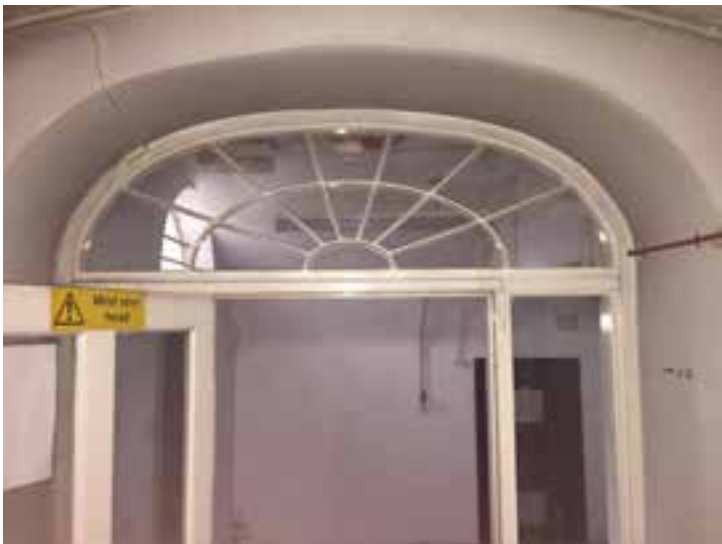
View of fan light over doorway under entrance steps
