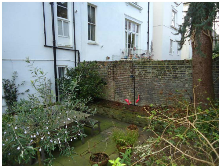
Photo 4 – Party fence wall with No.18
