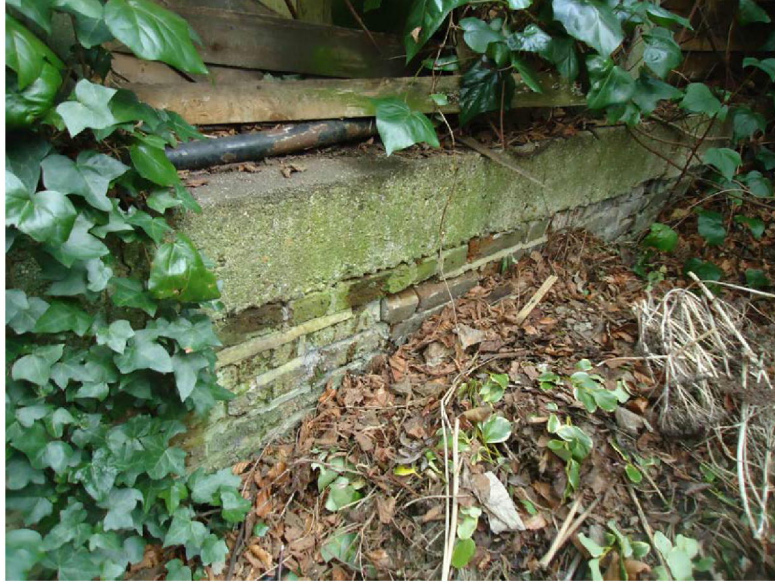
Photo 1 – Party fence wall to the rear
