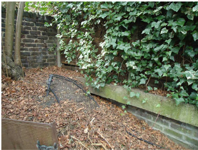
Photo 2 – Concrete plinth on the original wall to the rear elevation
