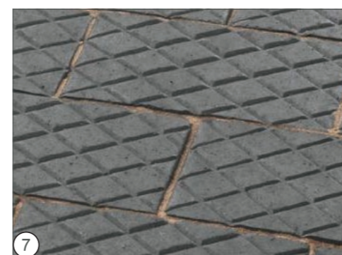
7 Brick to feature steps treads Supplier: Ketley Brick Product: Patterned Staffordshire Blue Pavers
