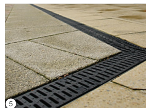
5 Channel drain with cast iron heels safe grating
