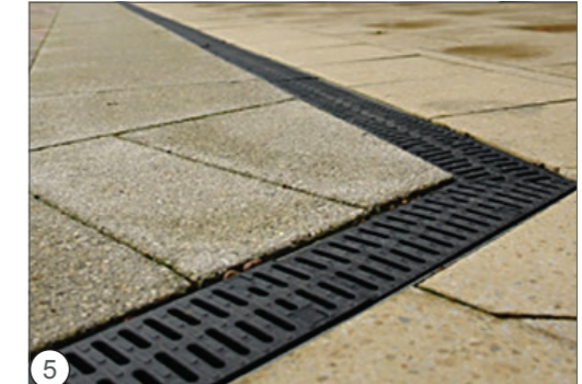
5 Channel drain with cast iron heels safe grating
