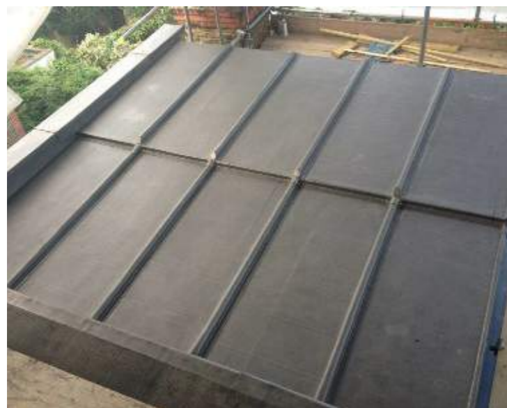
Image 23-24 Batten roll lead roof
