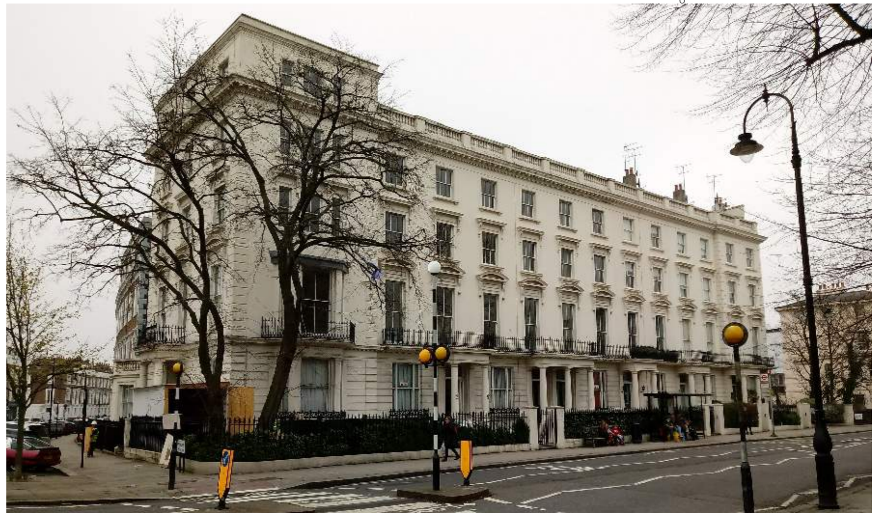
Image 07 Existing Building, street view
