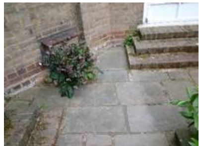
Trial pit 3 complete
