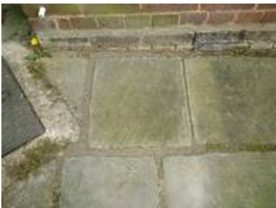
Trial pit 2 complete
