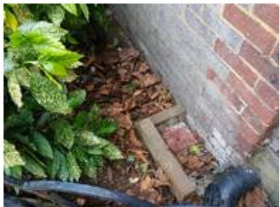
Trial pit 1 complete
