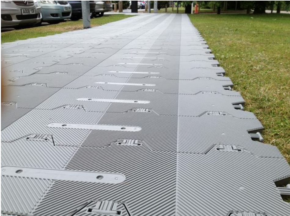
Figure 1 - Proprietary ground protection system
