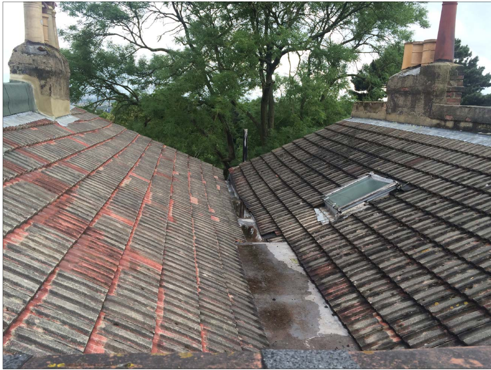
7 VIEW ROOF TOP
