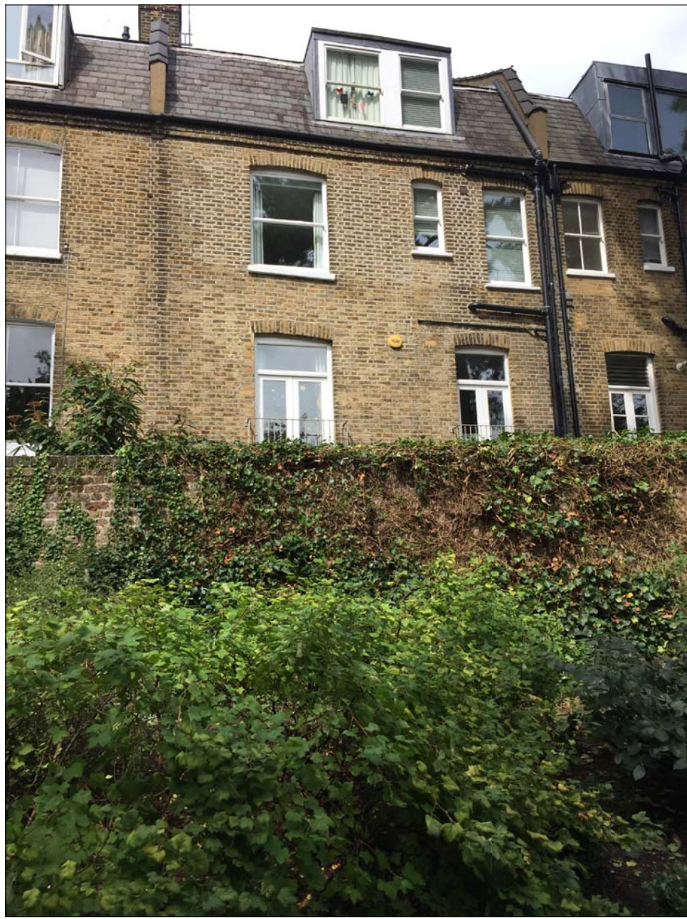
2 NEIGHBOR BUILDING VIEW
