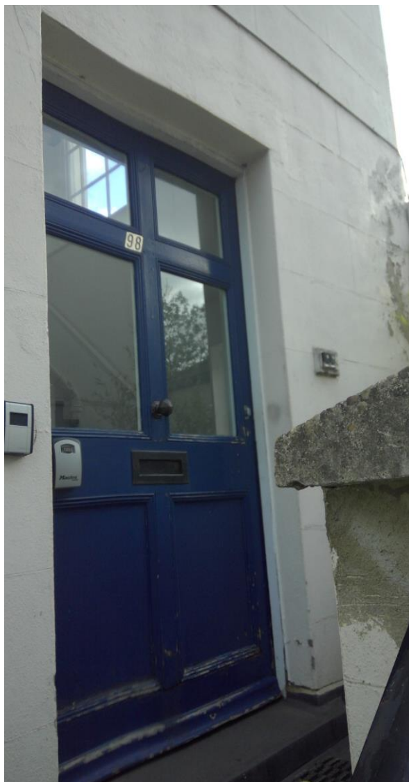
98 Fortess Road- Door Detail
