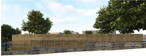
Ground Floor View - Existing
