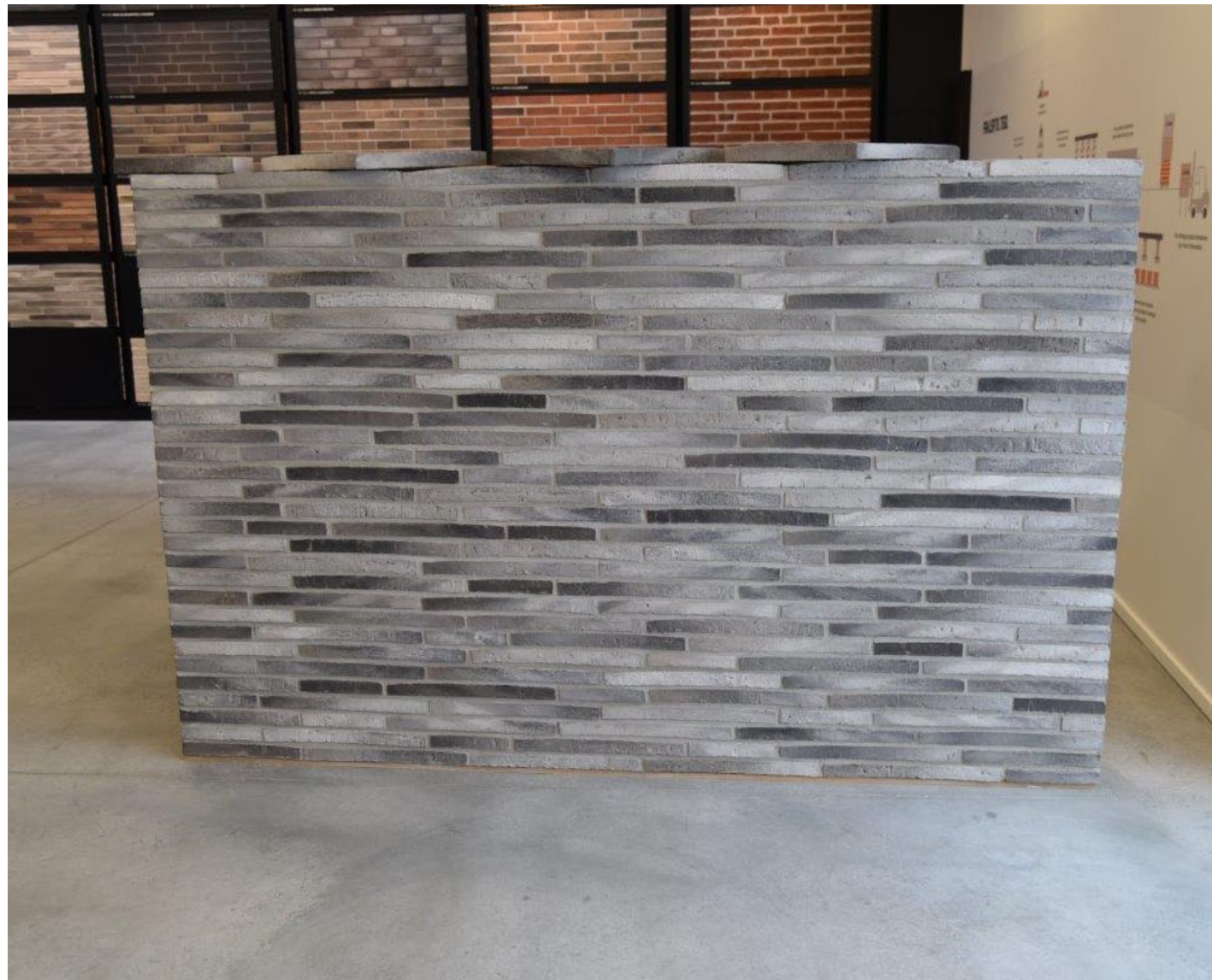
Large Brick Panel RT160 with Grey White mortar at Tegl factory in Aalborg, Denmark.
