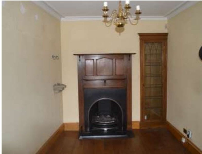
Figure 5.29: Arts & Crafts chimneypiece to front room in the 19th century extension (ground floor). Modern fire grate and fitted cupboard.
