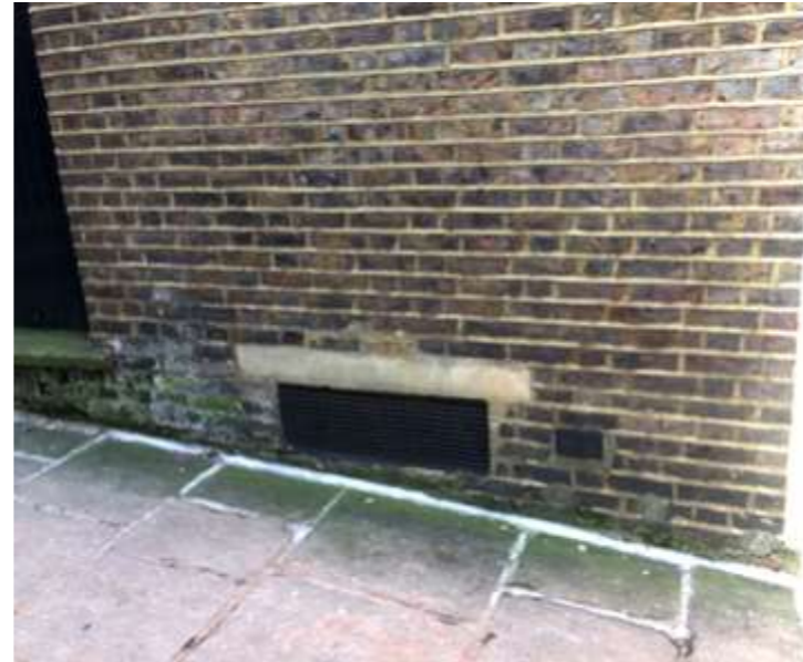
Figure 5.16: Basement window to existing rear bathroom, obscured by modern metal grille.
