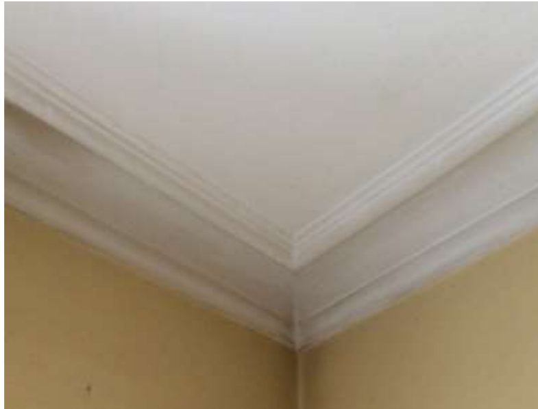
Figure 5.35: Historic cornice to front room of 19th century extension on the ground floor.
