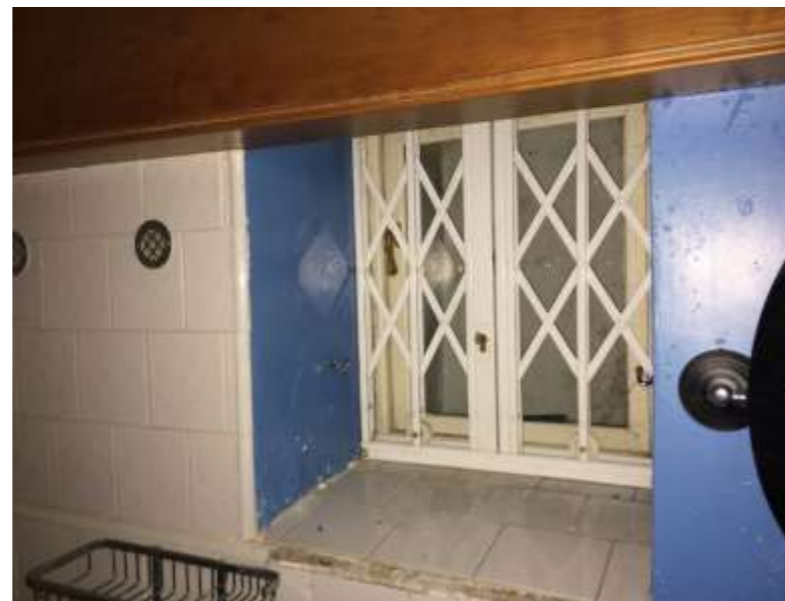
Figure 5.27: Existing window to rear bathroom at basement level. Existing water pipes are boxed in obscuring the window. Existing window likely dates to the 1940s.
