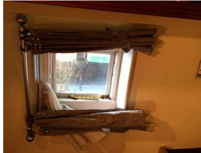
Figure 5.36: Mid 20th century casement window in ground floor bathroom.
