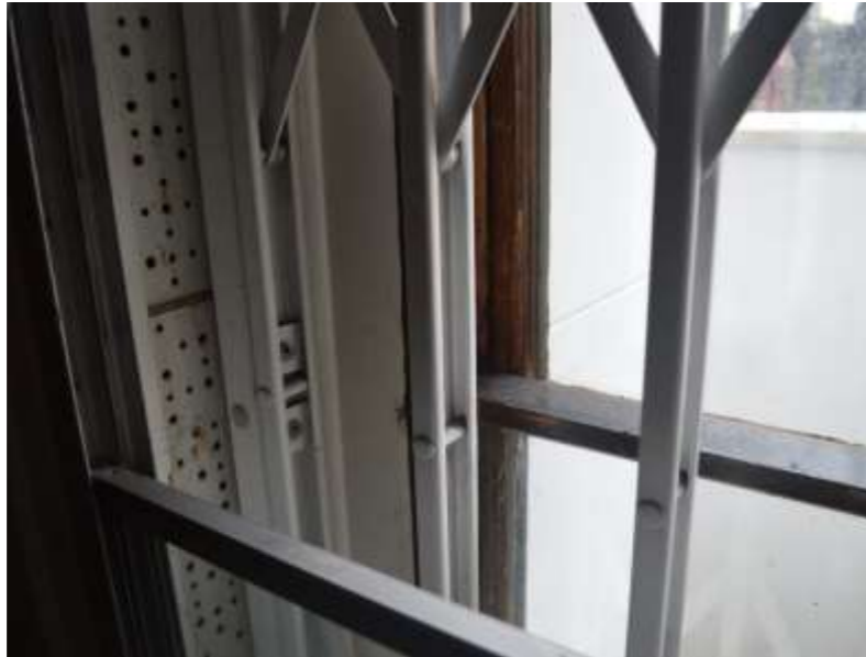
Figure 5.23: Window to front room at basement level, northern bay. Showing modern sash window, modern internal security grille, modern secondary glazing and perforated lining to window jamb.
