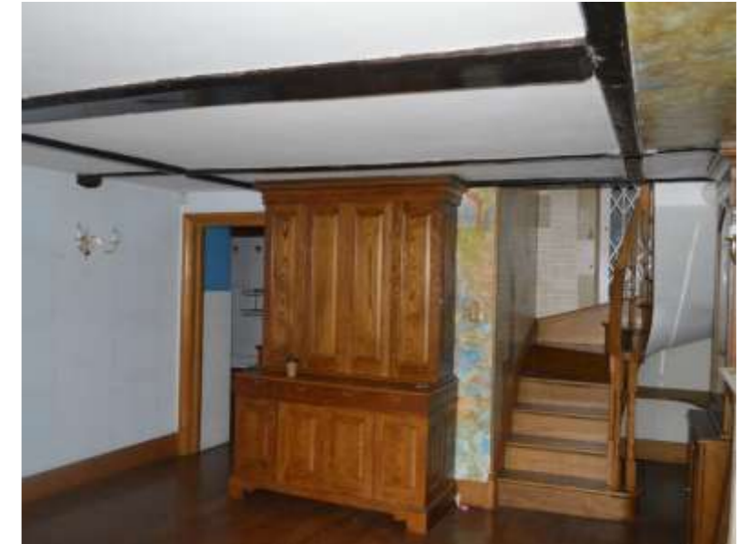
Figure 5.25: Front room to original house at basement level. Modern staircase, floorboards and door architrave. The main ceiling beam above is roughly chamfered in a Tudor manner and is likely a later affectation. Given their relationship to the modern ceiling surface the visible beams and joists may be fakes.
