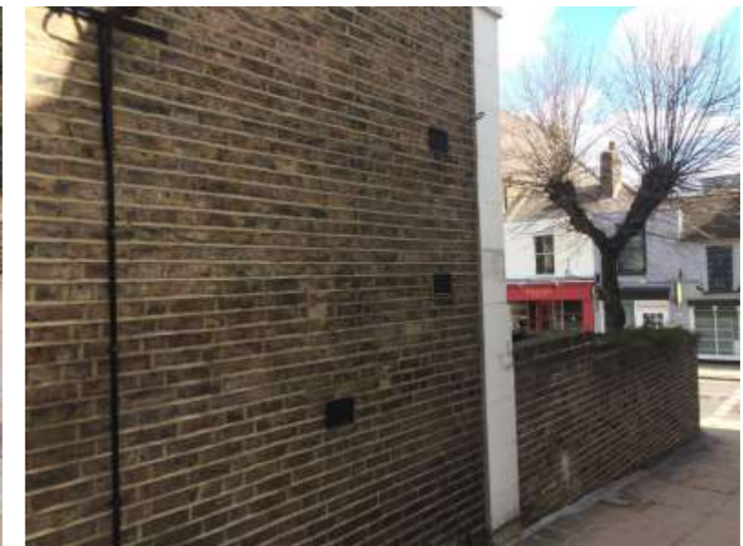
Figure 5.15: Southern (flank) elevation of No. 1 showing a number of grilled vents in the side wall.
