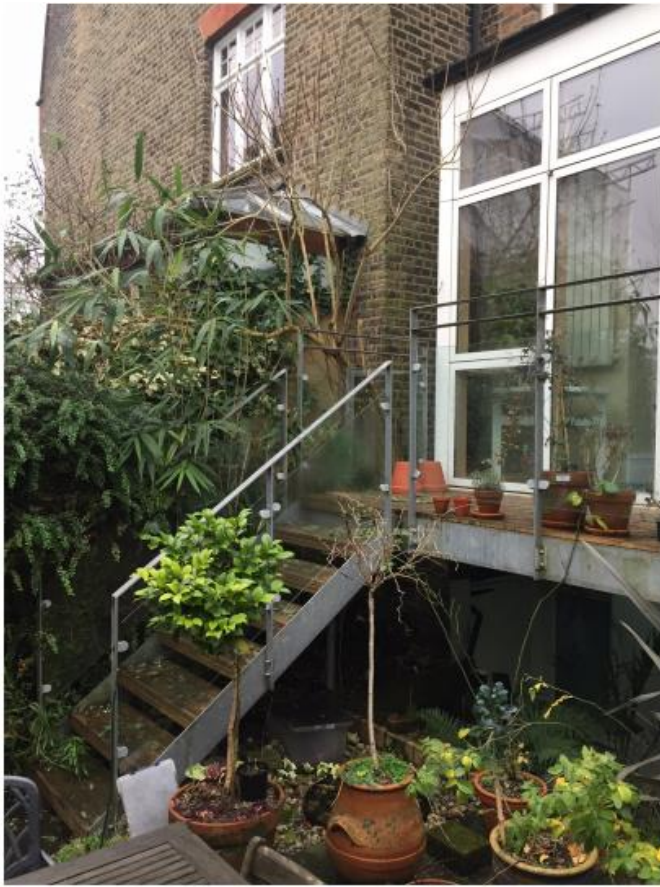
Below: Rear view from within the rear garden
