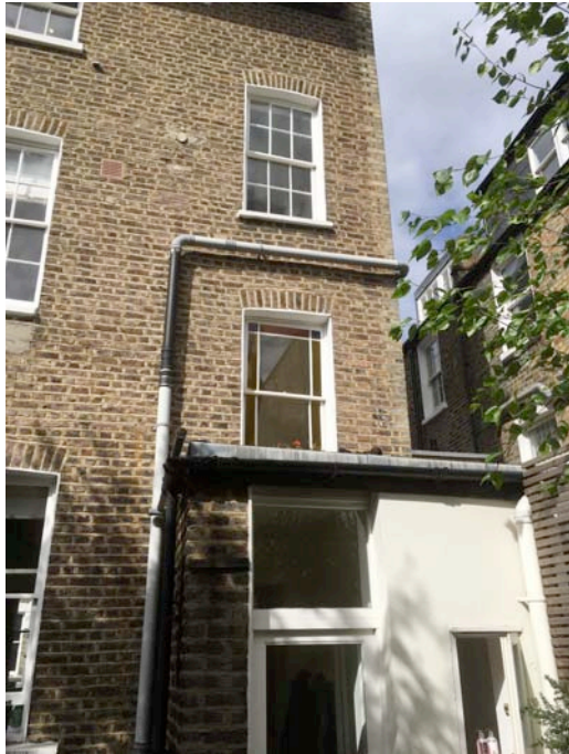
Rear elevation- closet wing showing rear door and WC window, proposed extension location
