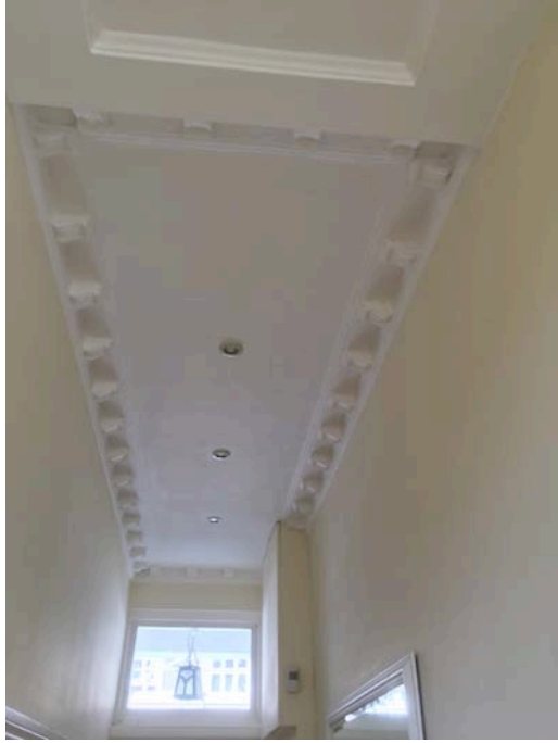
Ground floor- cornice to hall
