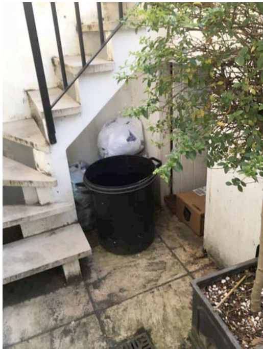
Front light well- existing stair and vault door
