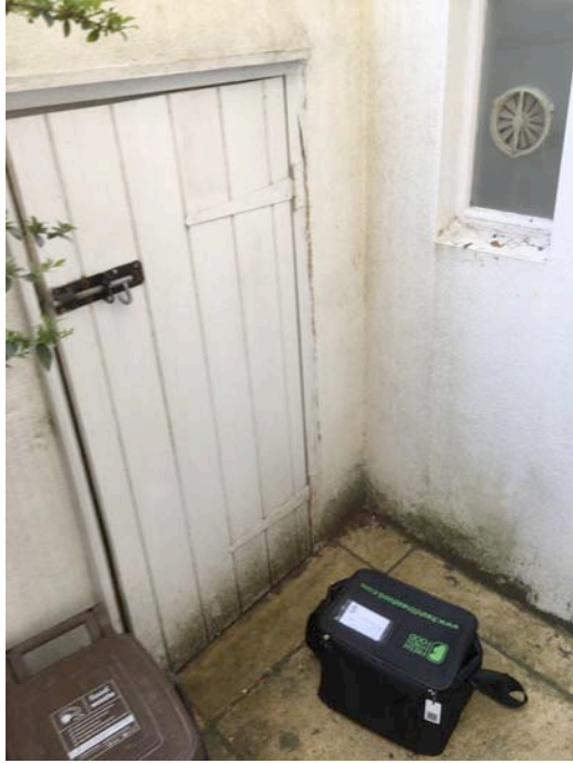
Front light well- existing vault door
