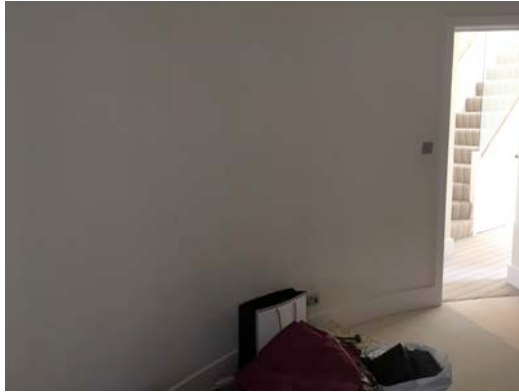
Second floor- curved wall
