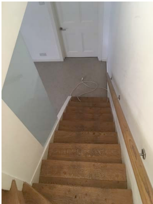
Lower ground floor- stair balustrade
