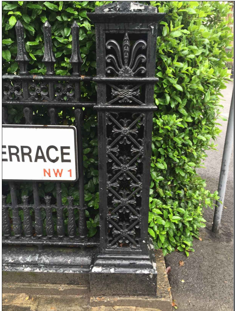
D-2 Photograph of existing open work box standard posts on cast iron base
