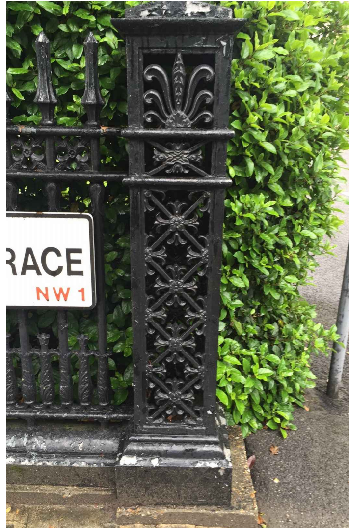
D-1 Photograph of existing open work box standard posts on cast iron base
