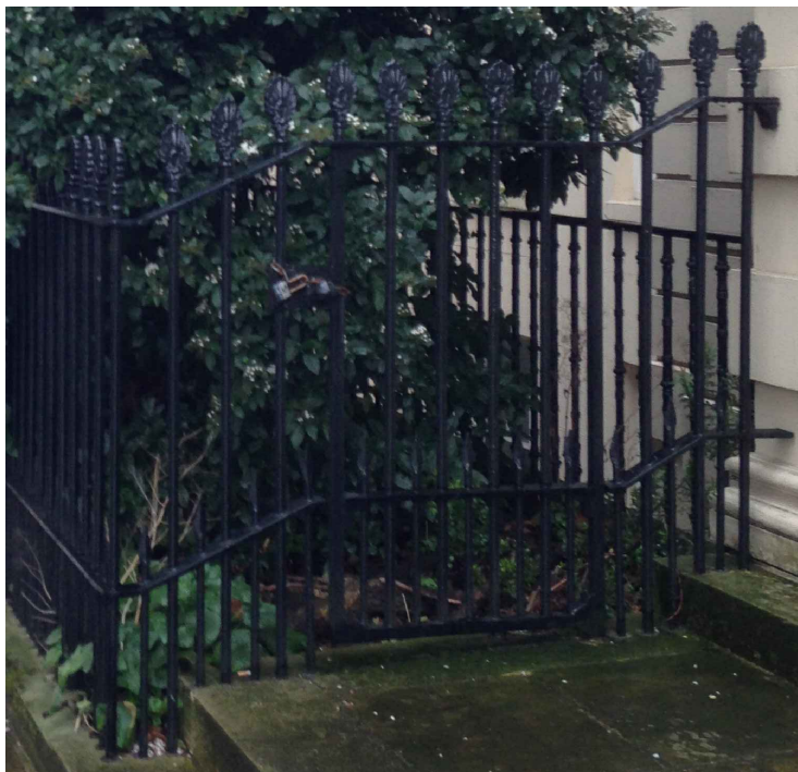
4 Photograph of existing RL.09 Railings with service gate and example of level change
