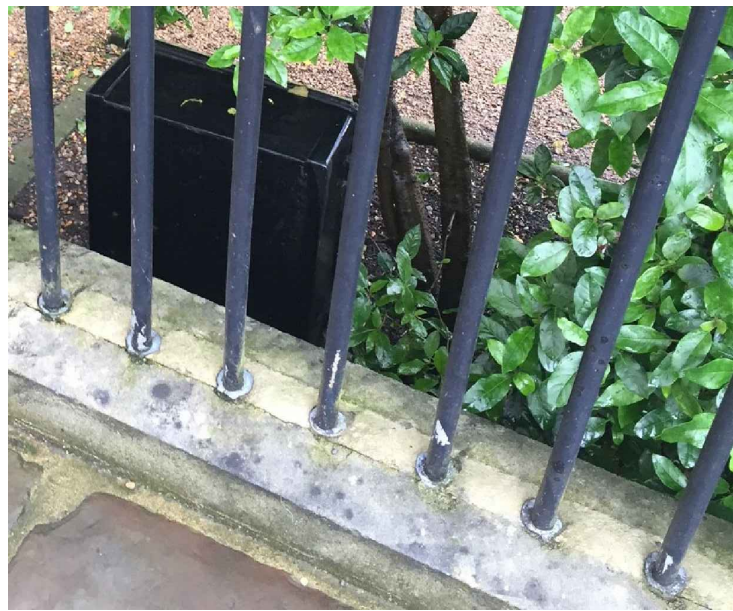
2 Photograph of existing railings led into stone plinth
