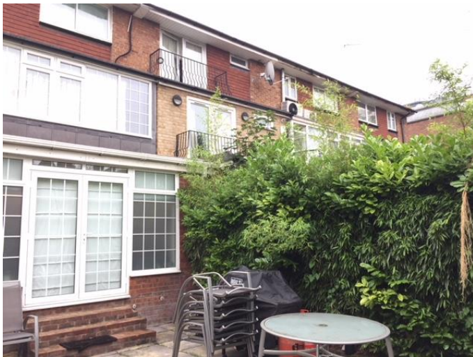
Photo 4 (above): Rear elevations of 14D, 14C, 14B and 14A Avenue Road
