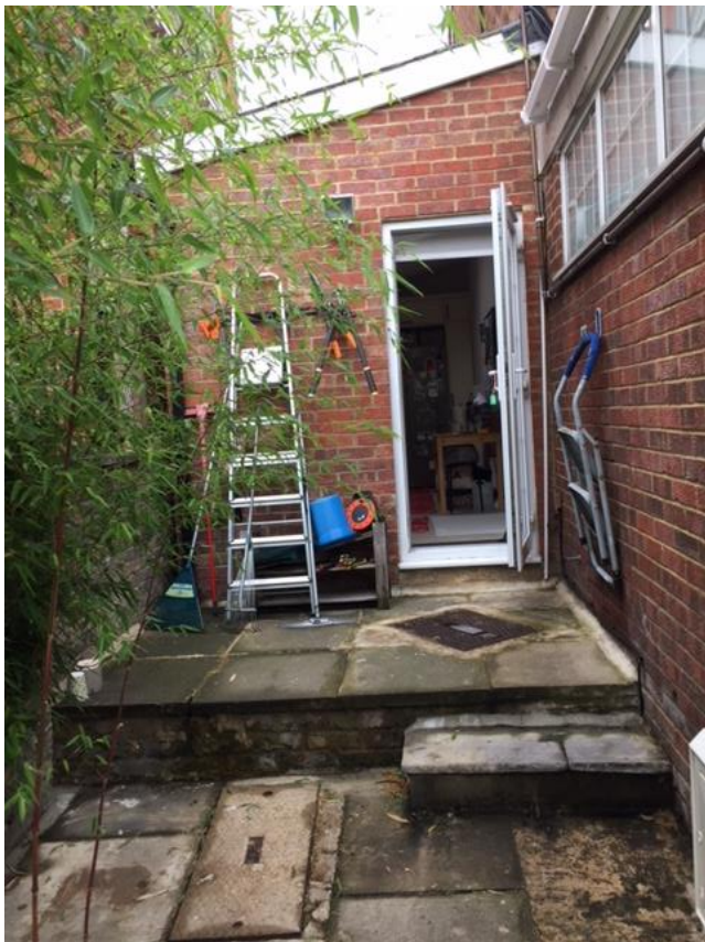
Photo 2 (above): Existing side and rear extensions at 14D Avenue Road
