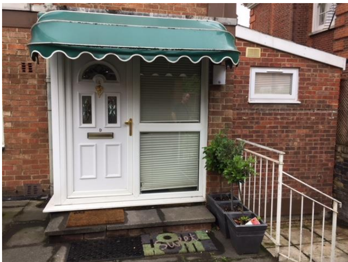
Photo 5 (above): Existing front porch and side extension at 14D Avenue Road
