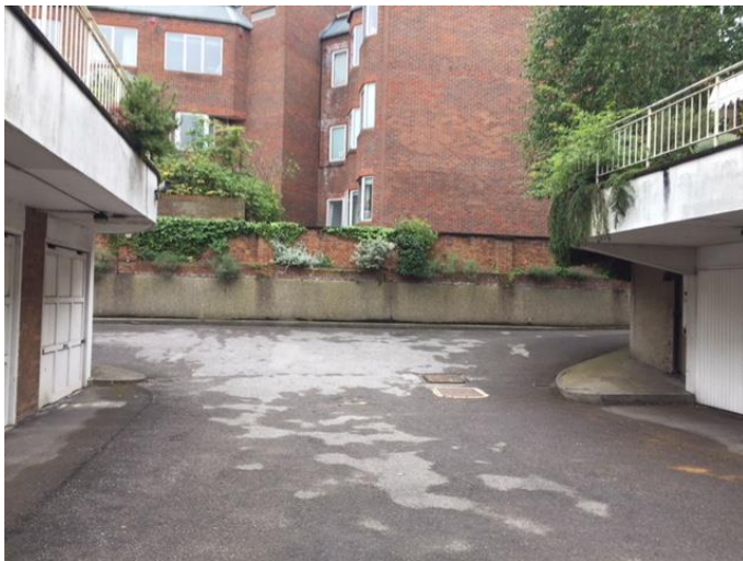
Photo 7 (above): Existing garages at basement level (looking south-east)
