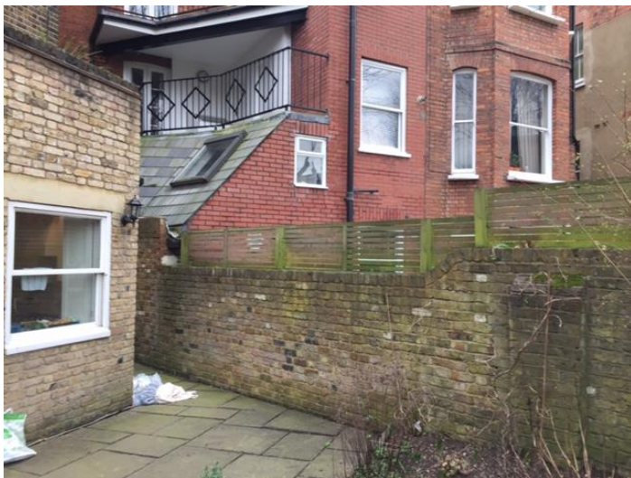
Photo 4 (above): Relationship between existing rear extension at 13a Crossfield Road and 37 Adamson Road to the south
