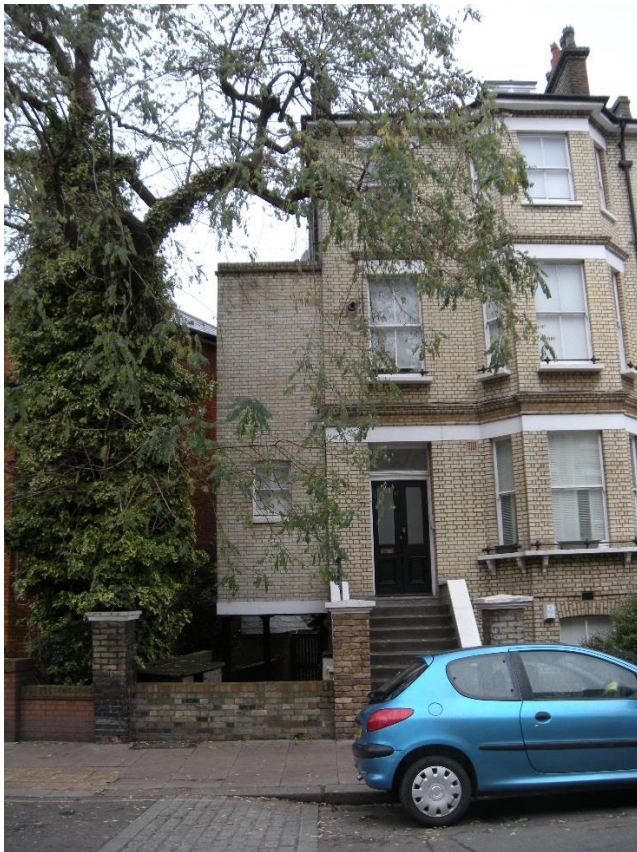
Photo 7 (above): Front elevation of 13 Crossfield Road
