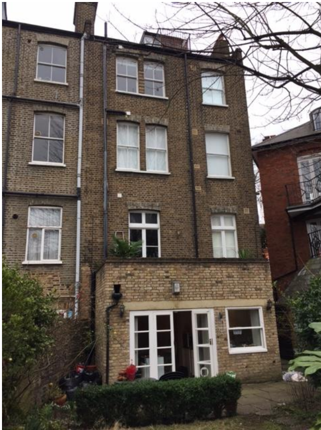
Photo 1 (above): Rear elevation of 13 Crossfield Road
