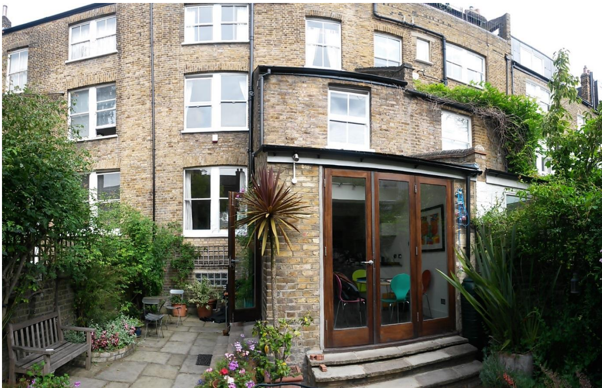
Photo 7 (above): Rear elevations of Nos. 54, 56 and 58 Croftdown Road
