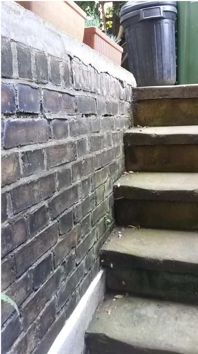
Photo 3 (above): Front steps leading to existing basement at 56 Croftdown Road
