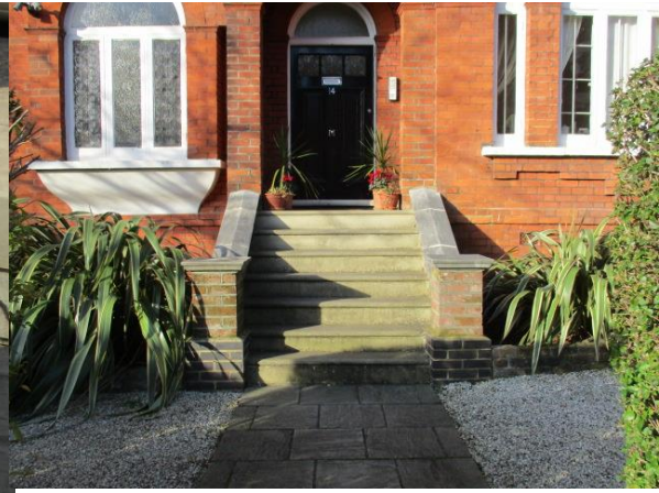
View of steps
