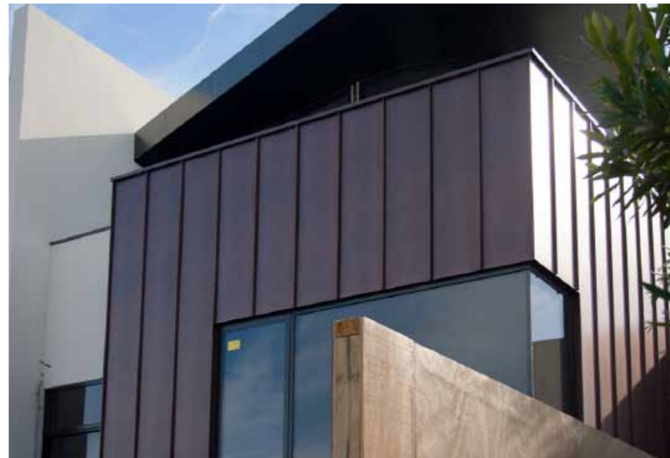
Dark copper colour standing seam zinc finish
