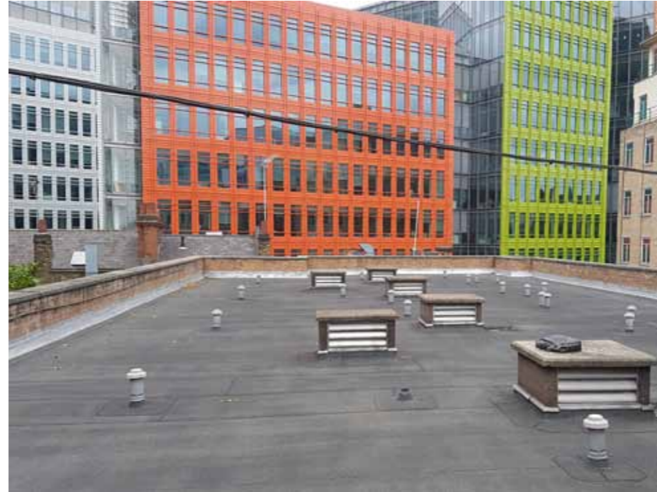
45 New Compton Street, Existing Rooftop
