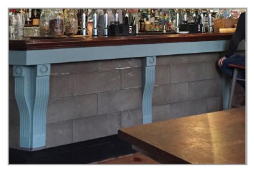
We will be stripping out the tiles to reveal the original wood which we will restore, sanding down the existing corbels.
