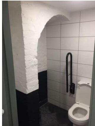
Photograph 2 – brick arch to be retained
