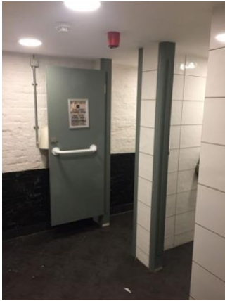
Photograph 1 - exposed brick work to be retained
