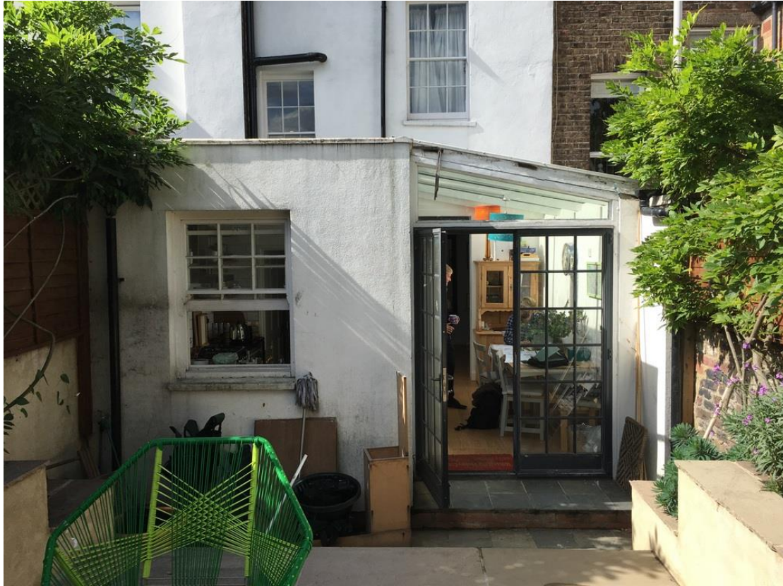
Figure 3: Rear elevation and rear extension to No. 4 Leverton Street.
