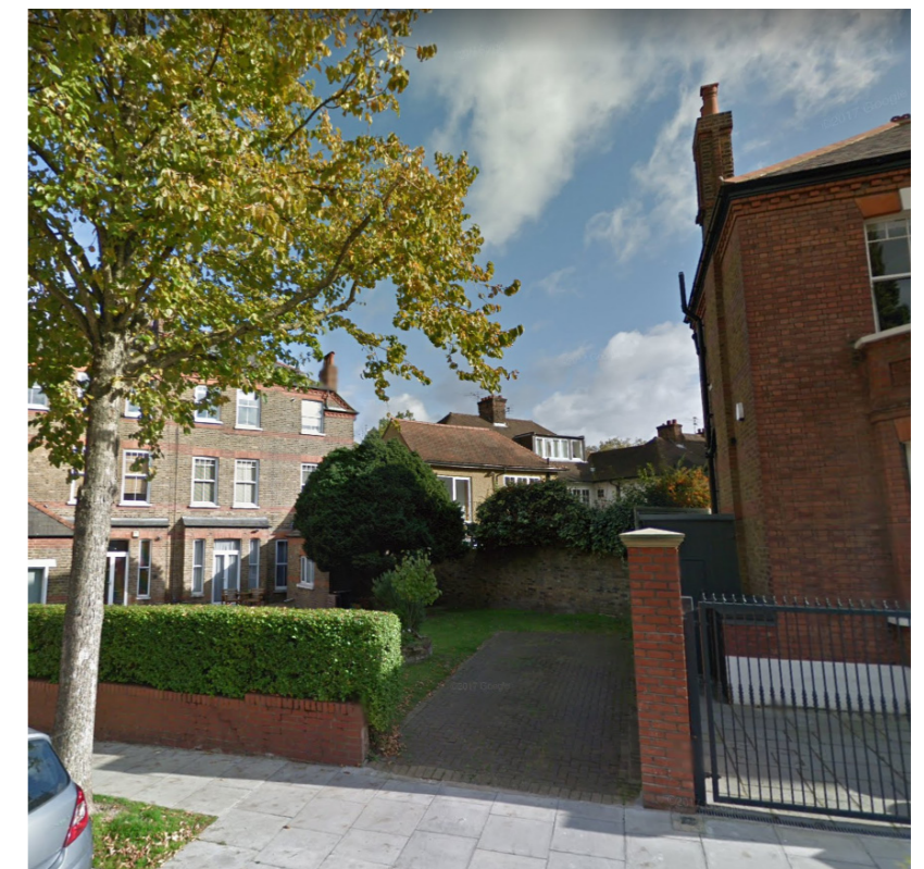
Rear view from Downside Crescent
