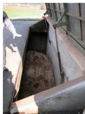
Figure 5: Pit storage system
