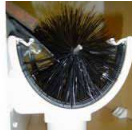
Fig 8 - Suitable gutter guards (2 types shown above) should be fitted to ensure that leaf drop from adjacent trees does not block new guttering leading to potential pressure for tree works.
