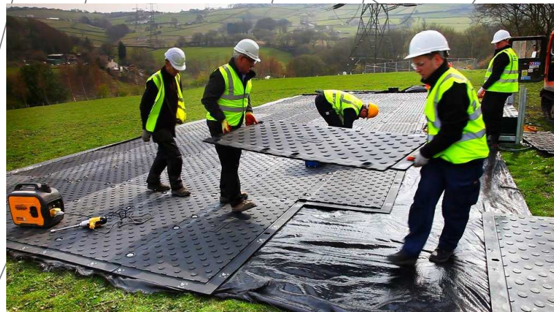
Temporary Ground Protection
