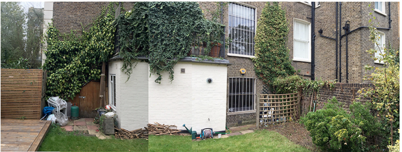
VIEW OF REAR ELEVATION TO LOWER GROUND FLOOR OF 22 WINCHESTER ROAD
