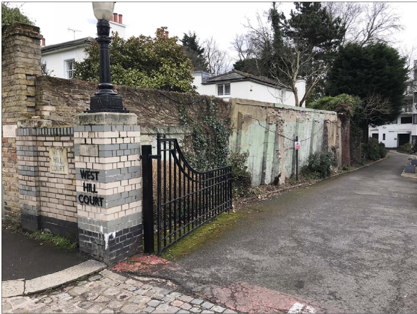
PHOTOGRAPH OF WALL, WEST HILL COURT ELEVATION
