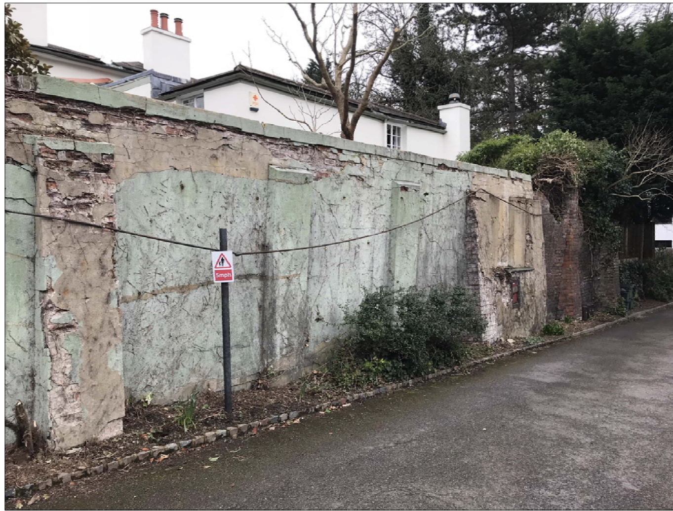
PHOTOGRAPH OF WALL, WEST HILL COURT ELEVATION
