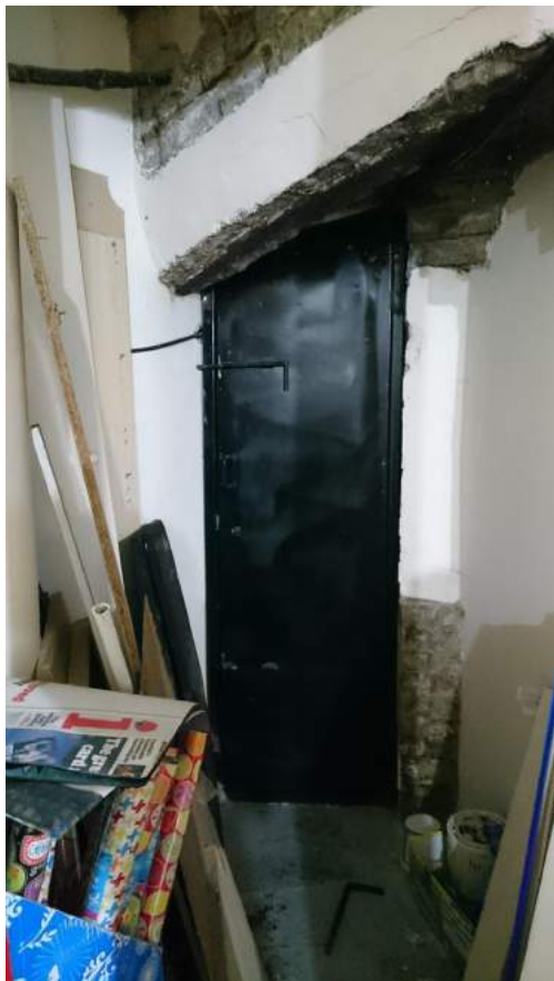
Figure 10 . View of basement door to under-street vault (not inspected).
