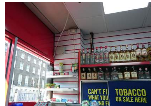
Figure 31. The suspended ceiling is cutback from the glazing and remains high enough to not interrupt the visual field at the proposed transom window level.
