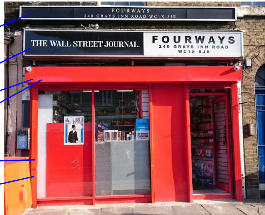
Figure 13. View of shopfront as taken on 6 February 2018 with contravening elements annotated.
