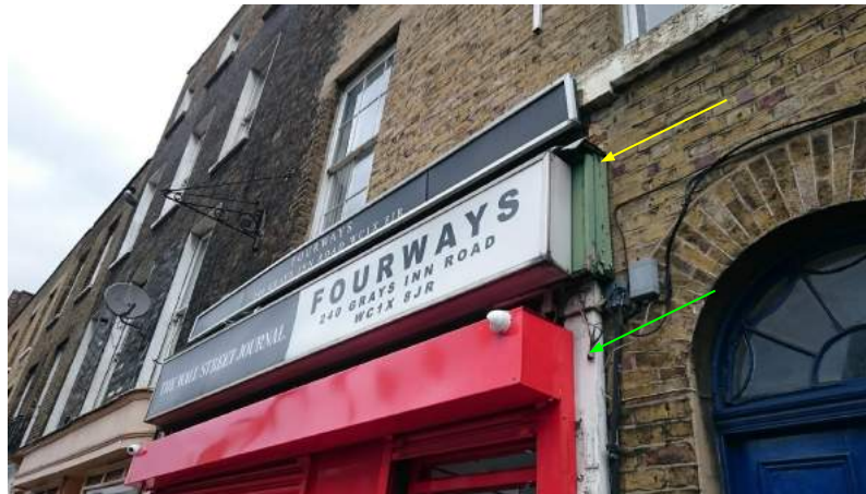
Figure 30 . Existing fascia (yellow arrow) and pilaster (green arrow) to be revealed and restored.
