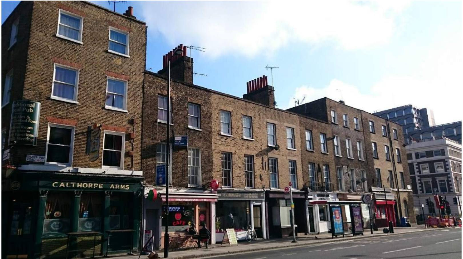
Figure 4. View of nos. 240 - 252 Gray's Inn Road, a terrace of Grade II Listed houses with 19th c. shops. No. 240 bookends the terrace with the Calthorpe Arms Public House (no. 252).
