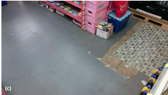
Figures 18 (a) - (d). Views of the floor to the shop. Note (b) also shows a small area of the wall finish and the slot bar elements to the wall shelving system. (c) and (d) also so a small reveal of the existing floorboards where the upper layer of gray lino has been lost.
