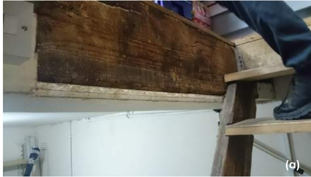
Figure 32 (a) - (b). Views of the staircase via the trap door from the shop to the basement store room. (a) Note the side face of the wider beam and two layers of plasterboard applied to the ceiling structure. (b) The rudimentary staircase in situ.
