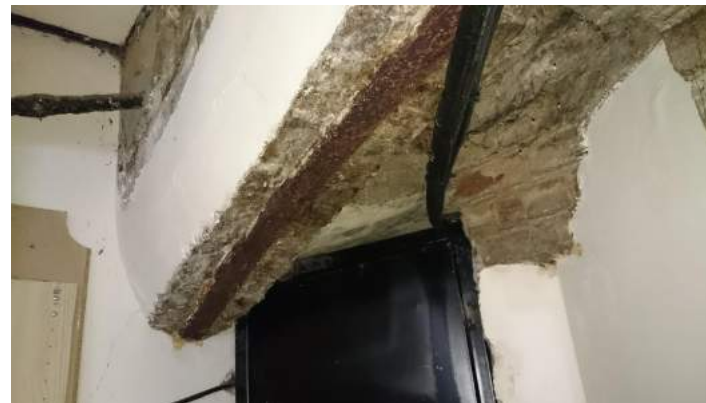
Figure 11. View of basement under-arch area with historic steel reinforcing band.
