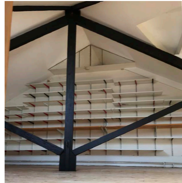
Timber structural beams across Third Floor
