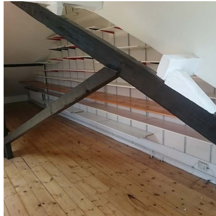
Timber structural beams across Third Floor
