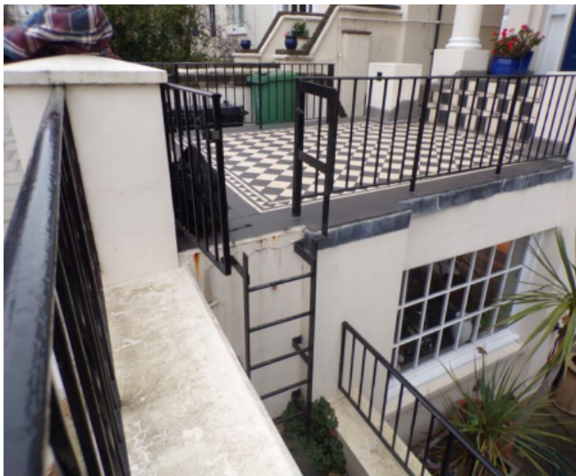
3) Tiled steps and existing pillar with coping stone
