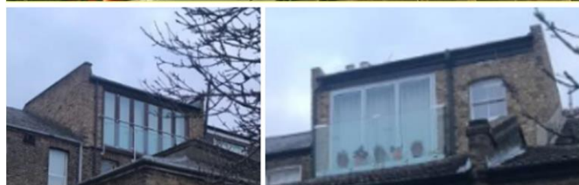
TOP: ROOF EXTENSIONS HAVE BEEN DEVELOPED AT NOS. 2-6, 9-11 BOTTOM: ROOF EXTENSIONS ARE FULL-WIDTH AT THE REAR AT NOS. 6 & 9
