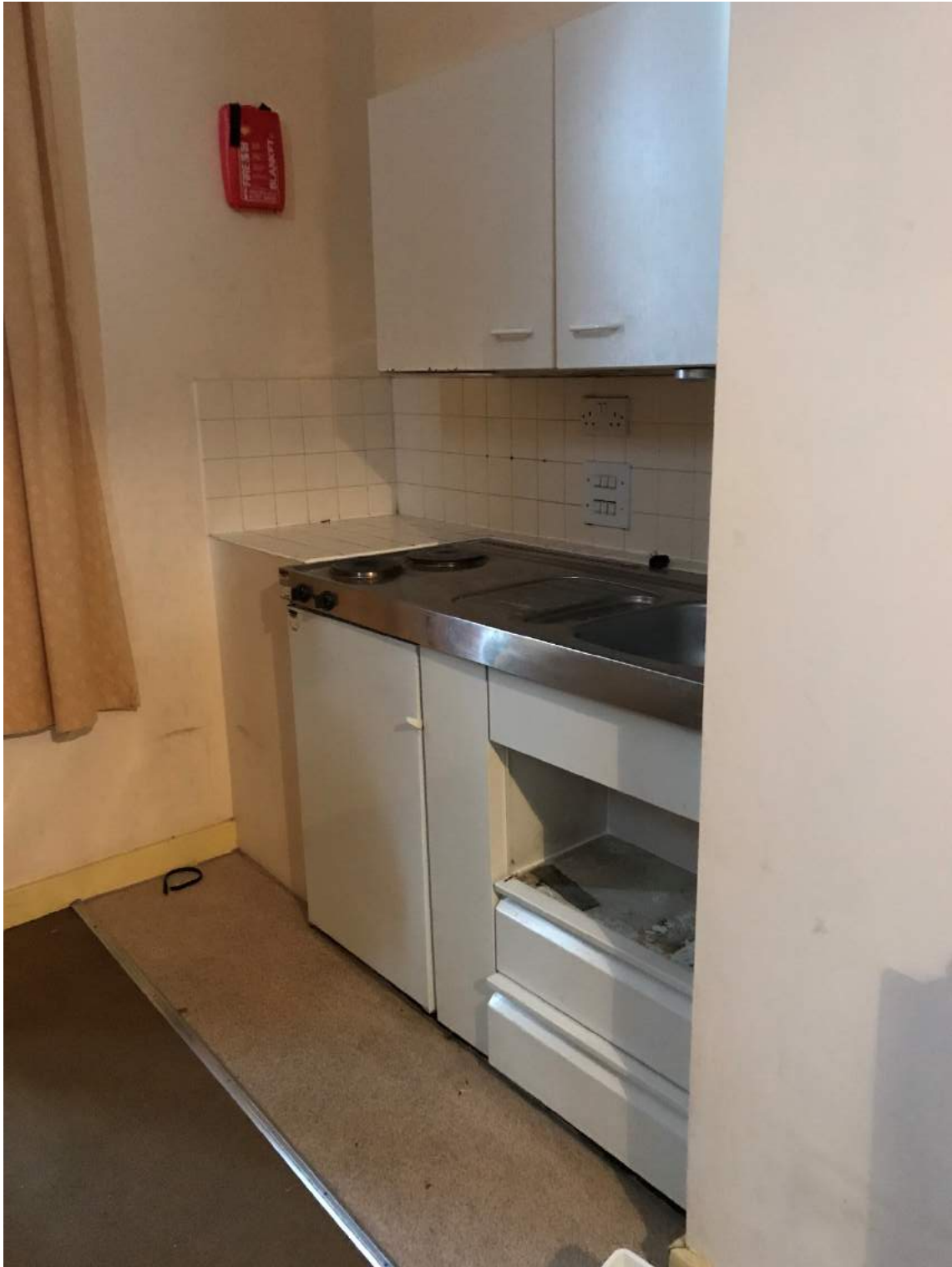
Figure 1: Typical kitchenette to be removed as part of Phase 1.
