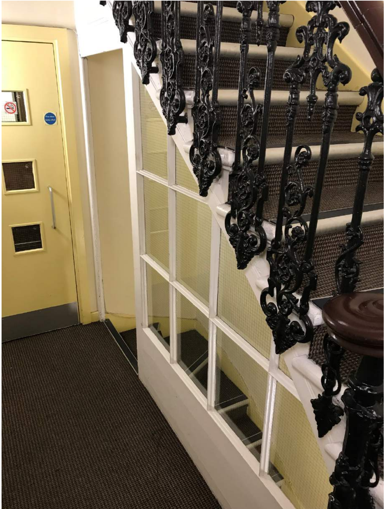
Figure 3: Stair and glazing below to be retained. Carpet to be removed as part of phase 1, and modern door proposed to be removed as part of phase 2.
