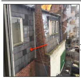
Material Sampled: Asbestos Cement slate tiles to roof elevations
