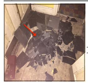
Material Sampled: Asbestos Cement roof slate debris to floor
