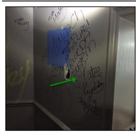
Material Sampled: Fibrous plasterboard to walls
