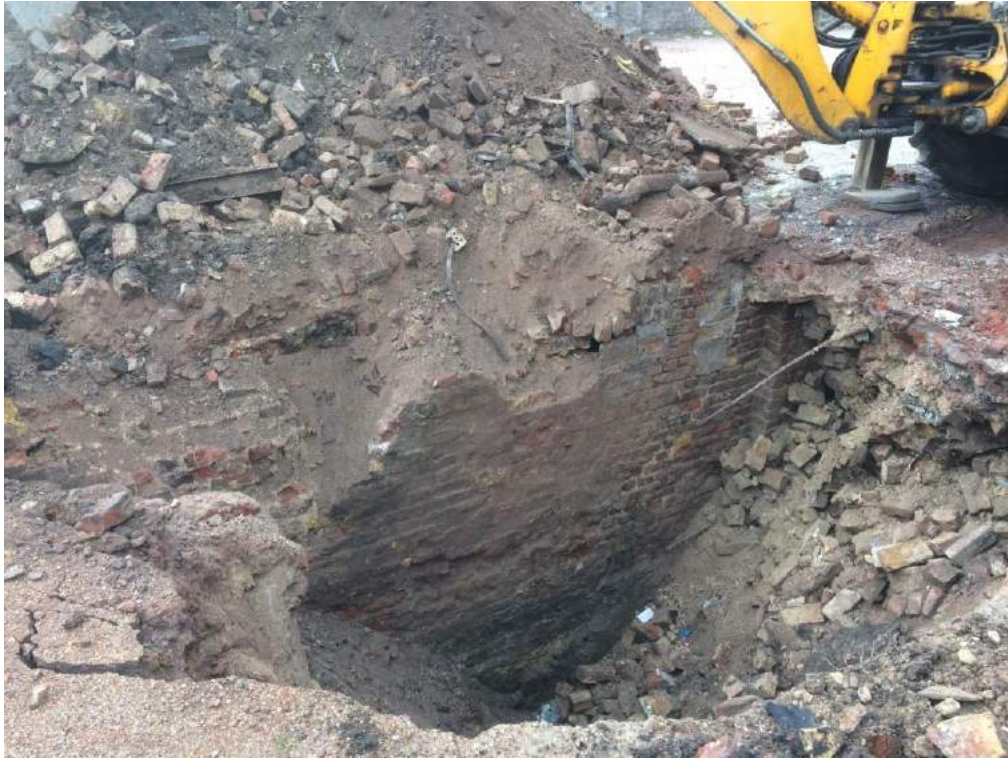
View to south west pit side
