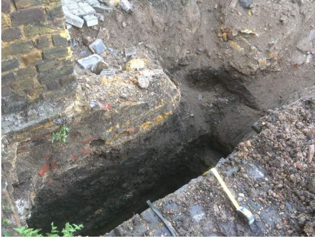
Sub-surface wall to north west of pit side
