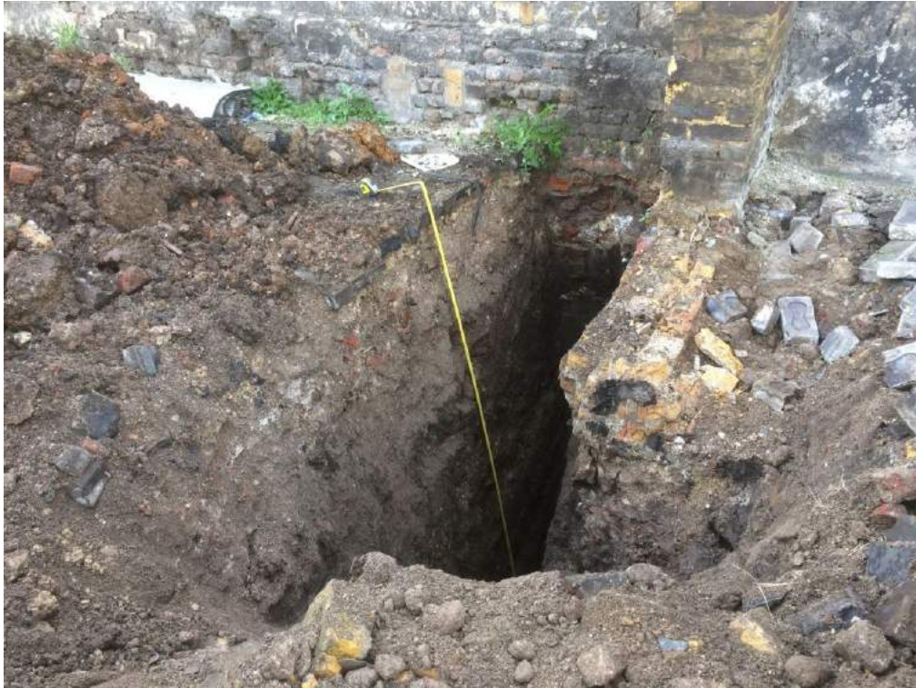
View towards south western site boundary wall with Gough Street
