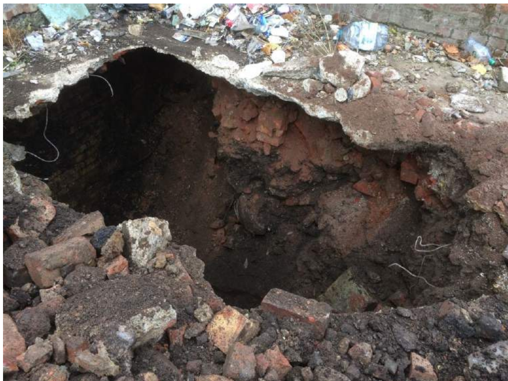
Loose backfill material visible in north west pit side.
