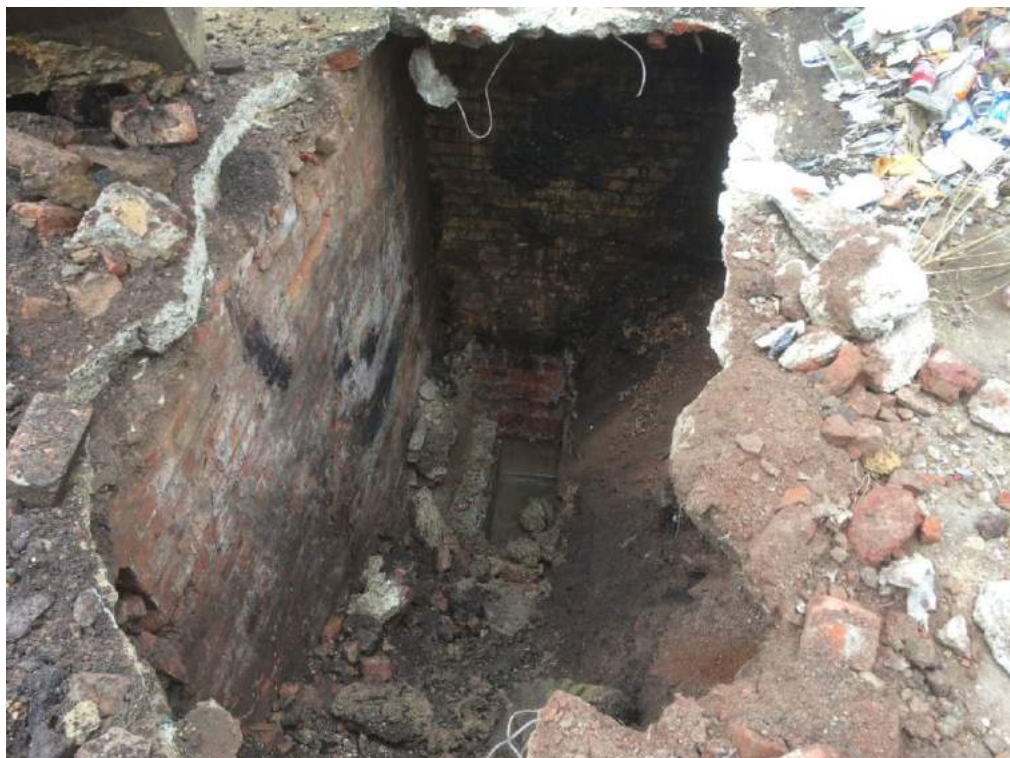
Photograph showing extent of site boundary wall and foundation profile at base of pit.
