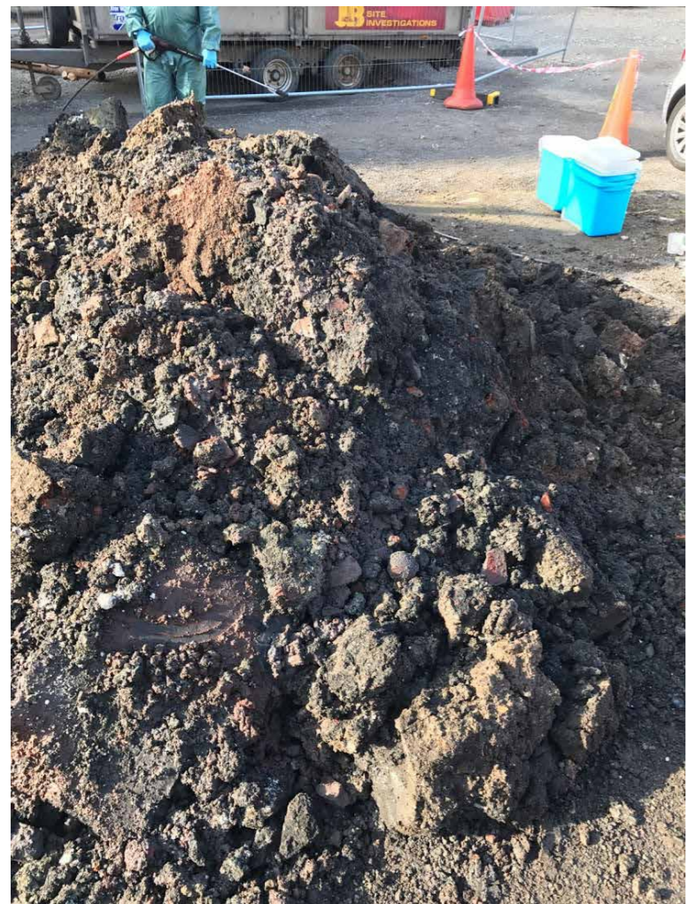
Spoil from TP10 - Note reddish brown deposit
