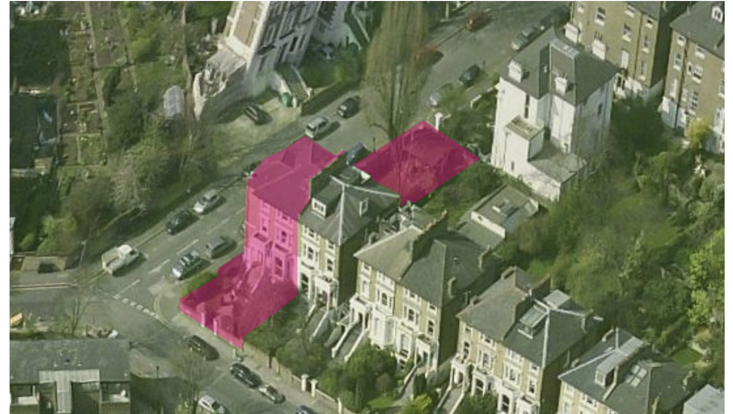
Ariel view to the West
