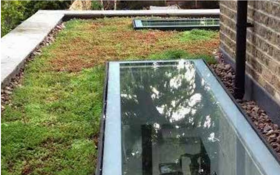
Extension Roof: Green Roof and Roof Lights
