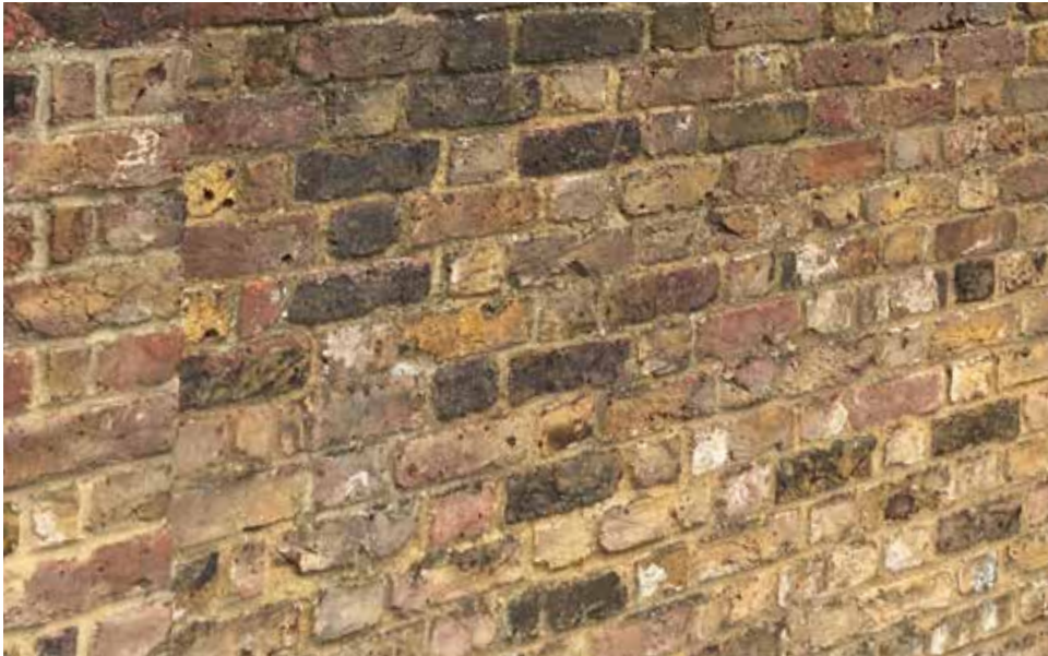
Extension Brick: London stock to match existing
