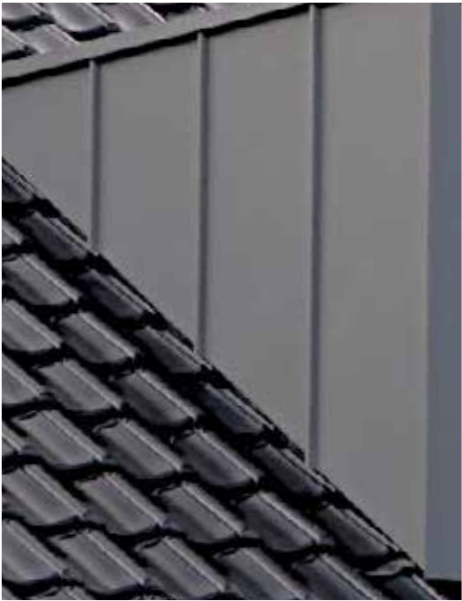
Zinc Clad Dormer Window
