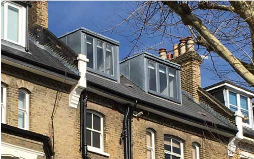
Zinc Clad Dormer Windows on Steels Road
