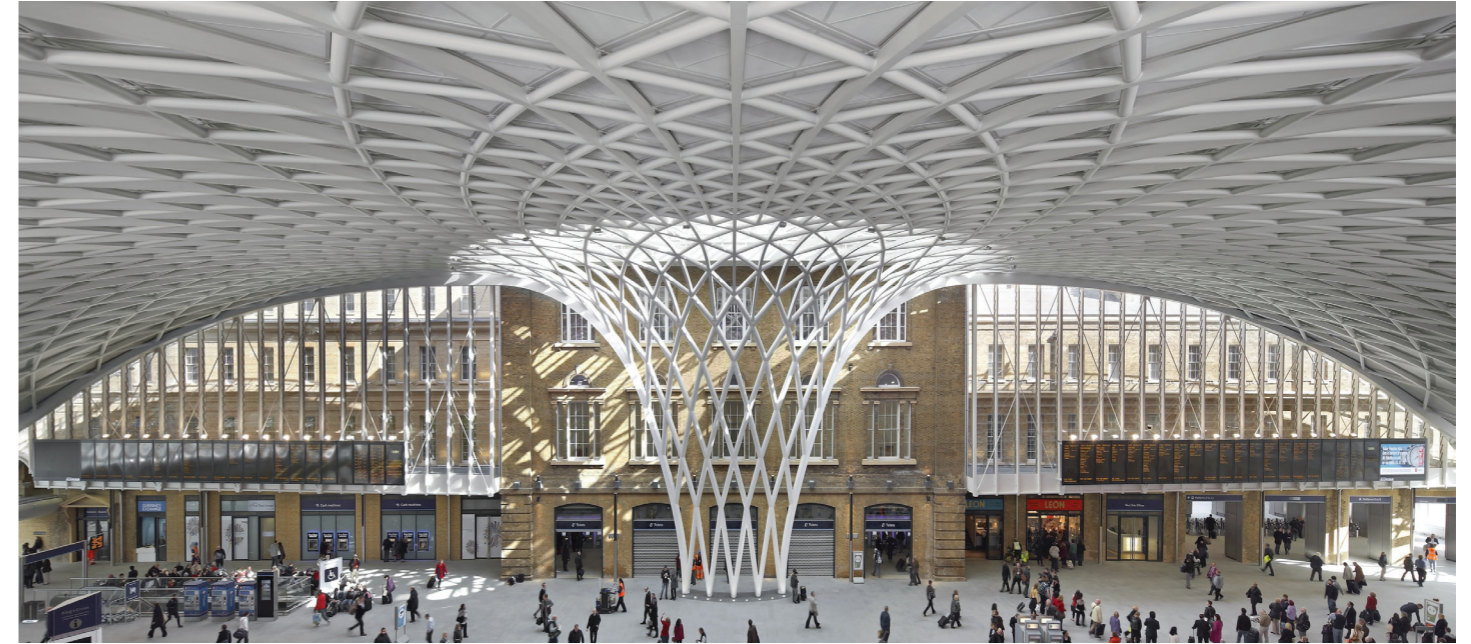
Fig. F.16 Photograph of the concourse showing the 'funnel' roof support structure in the centre
