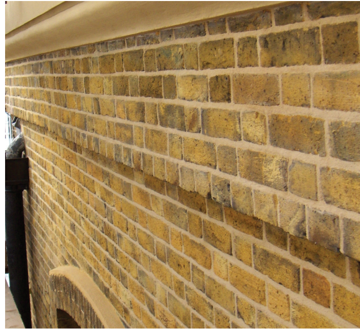
Fig. F.5 Good quality brickwork repair on the Western Range
