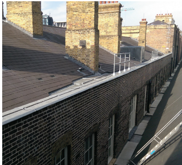
Fig. F.1 Western Range Key Clamp handrail
