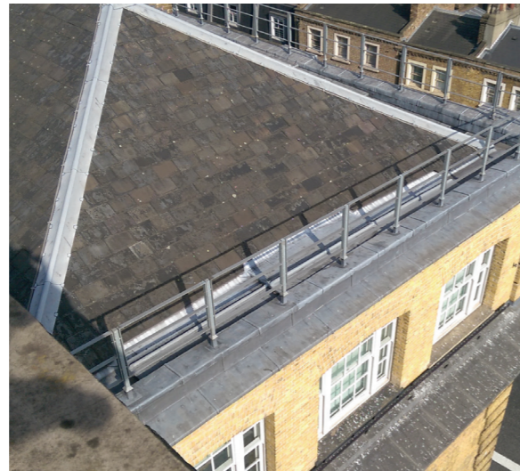
Fig. F.2 Eastern Range parapet handrail
