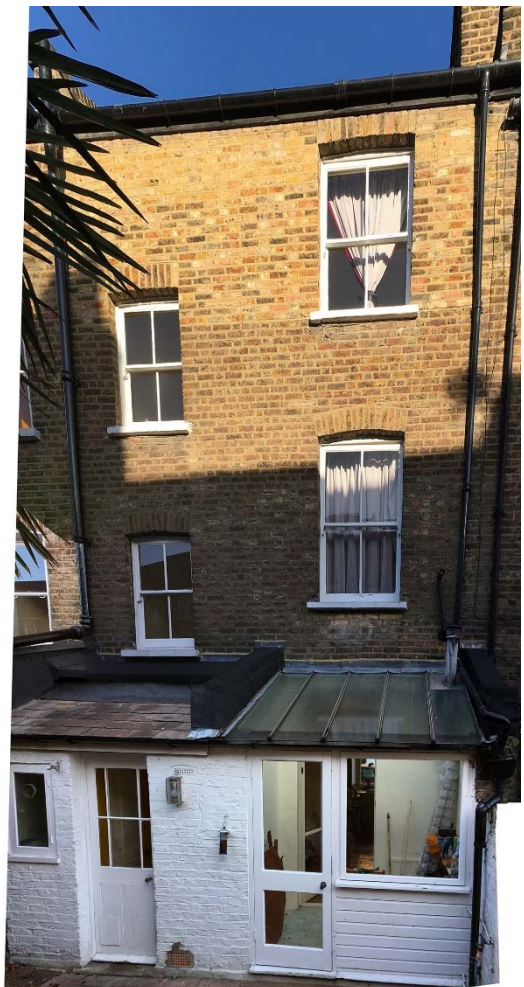
Rear elevation of 42 Chetwynd Road
