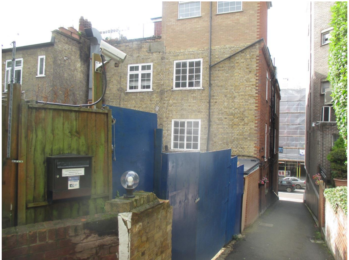
Image 5. View from the side passage towards Finchley Road.
